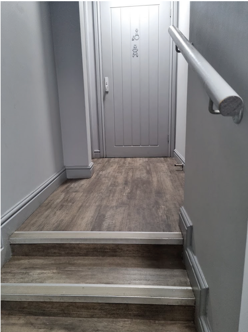
Figure 1 shows a toilet marked as accessible, but up steps. This shows that the toilet was tokenistic with no work to ensure it was accessible for disabled people to use.
